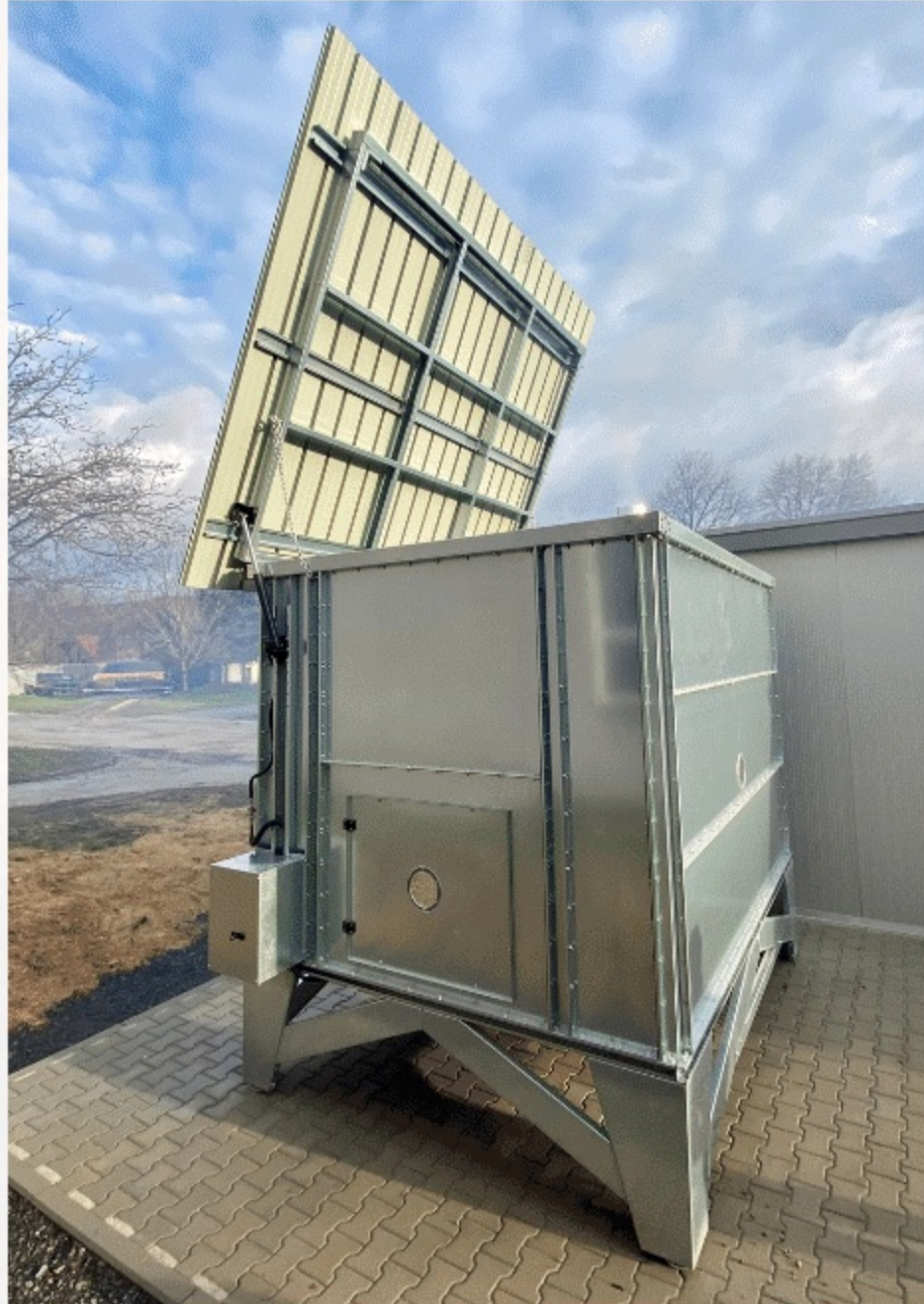
External tank for biofuels
